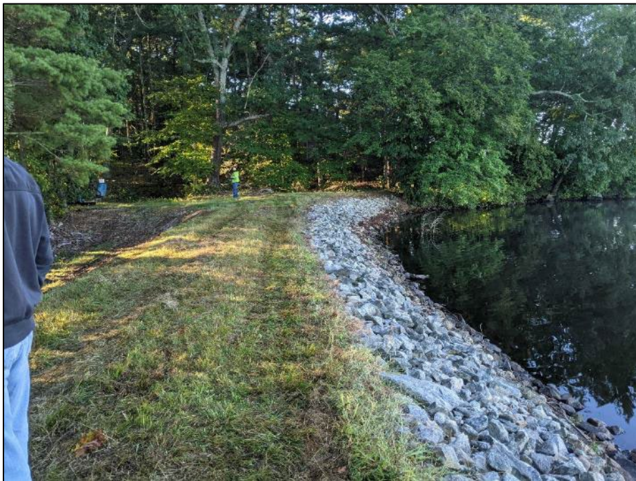
Photo No. 4.: Crest of the dam from study area looking right.
